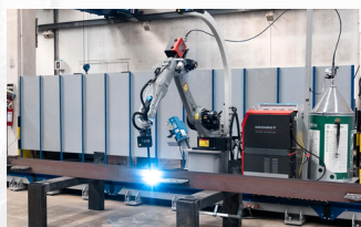
ROBOTIC WELDING OF BEAMS
